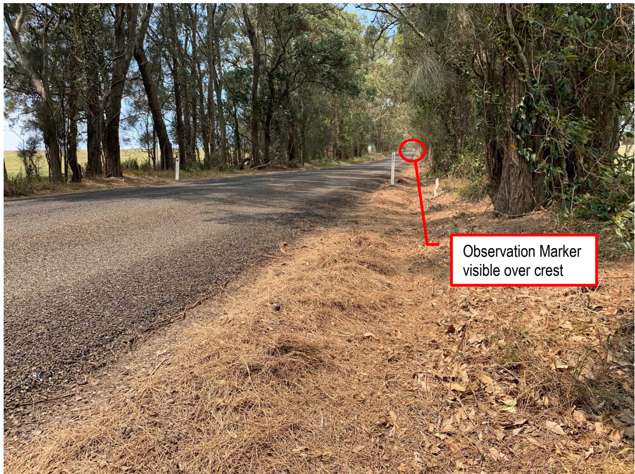
Figure 2 – Western Intersection – Looking East – SISD 317m
